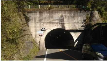
Sasago tunnel at Otsuki.
